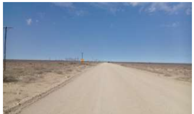
Photo 6: Road to Kronos substation
