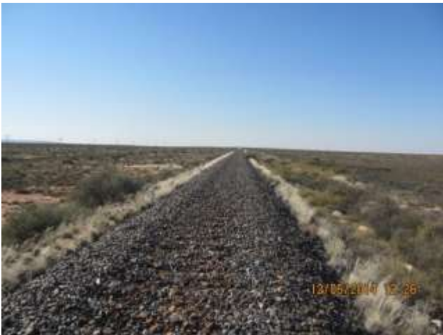
Photo 4: Decommissioned railway line
