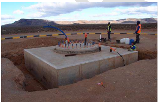
Photo 5: Completed MeerKAT foundation after stripping of formwork
