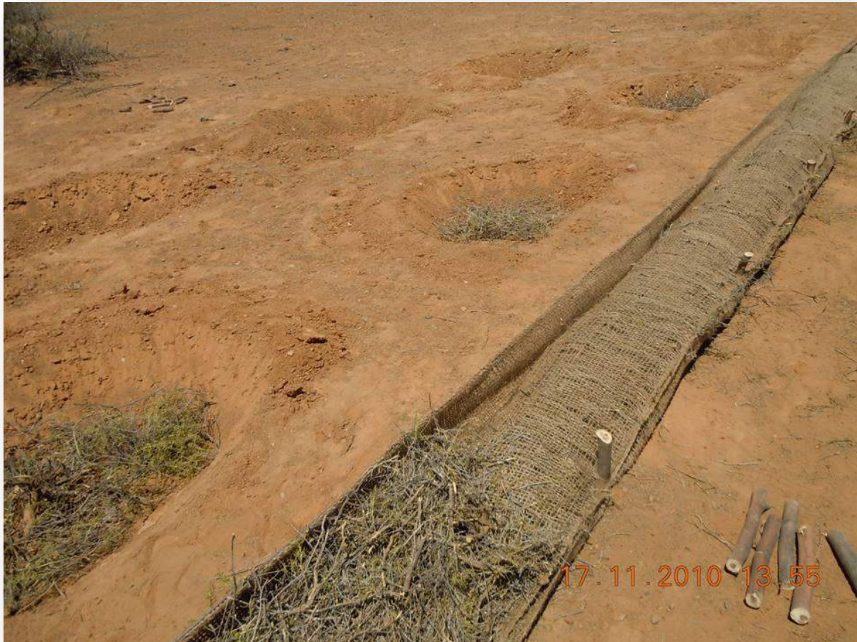
Figure 5-3: Prosopis brushwood used as pegs and filling for erosion control “sausages”, as well as mulch in hand dug mini-catchments
