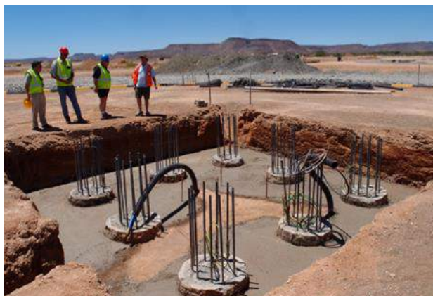
Photo 1: MeerKAT antenna foundation piles
