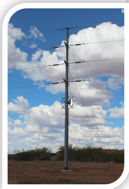
Figure 2-15: Steel monopole strain structure showing silicone rubber composite longrod insulator.
