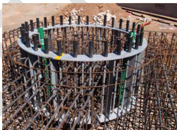
Photo 4: Pile cap reinforcement incorporating bolt assembly cage
