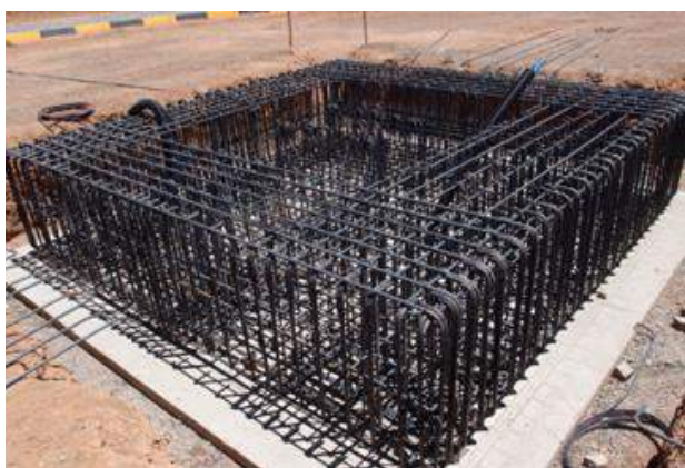
Photo 3: Pile cap reinforcement
