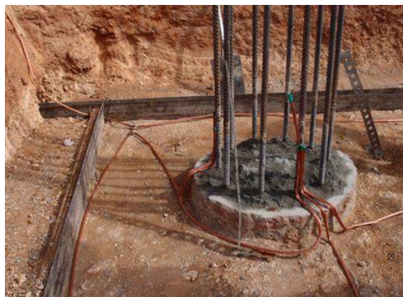
Photo 2: Earthing and lightning protection scheme
