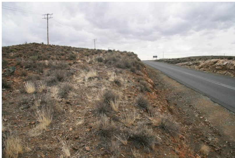
Figure 30: Road cutting through low hills in the Eastern Upper Karoo.
