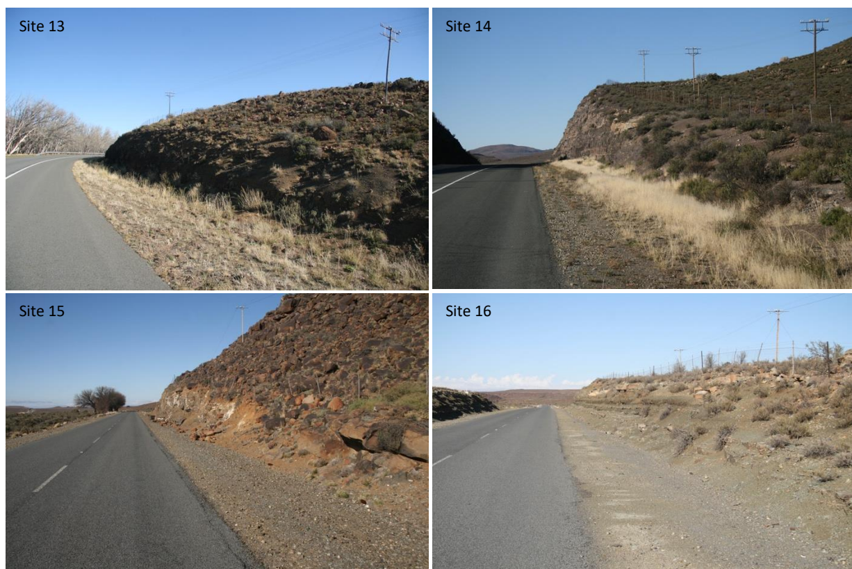
Figure 41: Instances on the underground section where trench where the trench cannot go over the cutting, but should be next to the road. (a) Site 13; (b) Site 14; (c) Site 15; and (d) Site 16 (see text for GPS co-ordinates).
