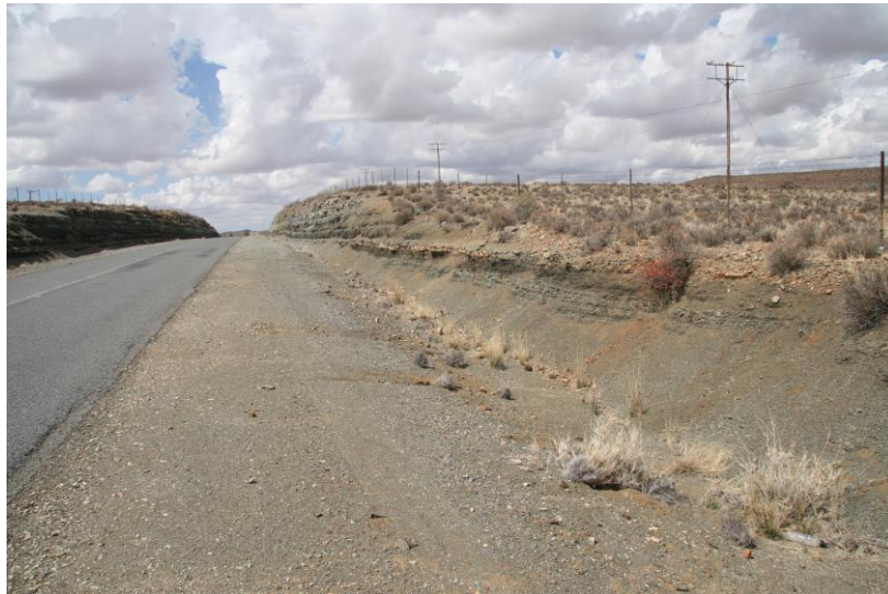
Figure 31: Road cutting through low hills in the Eastern Upper Karoo.
