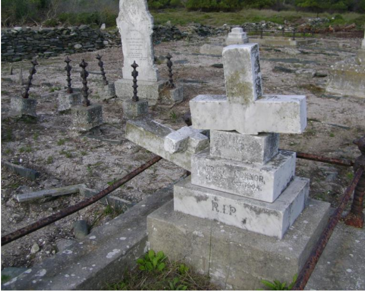
(b) Slanting of a tombstone on top of a grave... It has been broken.
