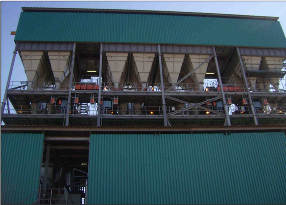
Plate 2.10: Retort feed bins above the retorts.
