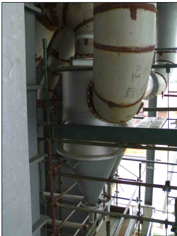
Plate 2.18: The cyclonic separator.
