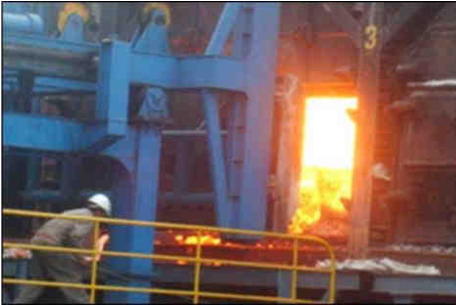
Figure 2.7: Pushing/charging machine opening coke oven door. View of heated coke cake in oven (Courtesy Sinosteel)
