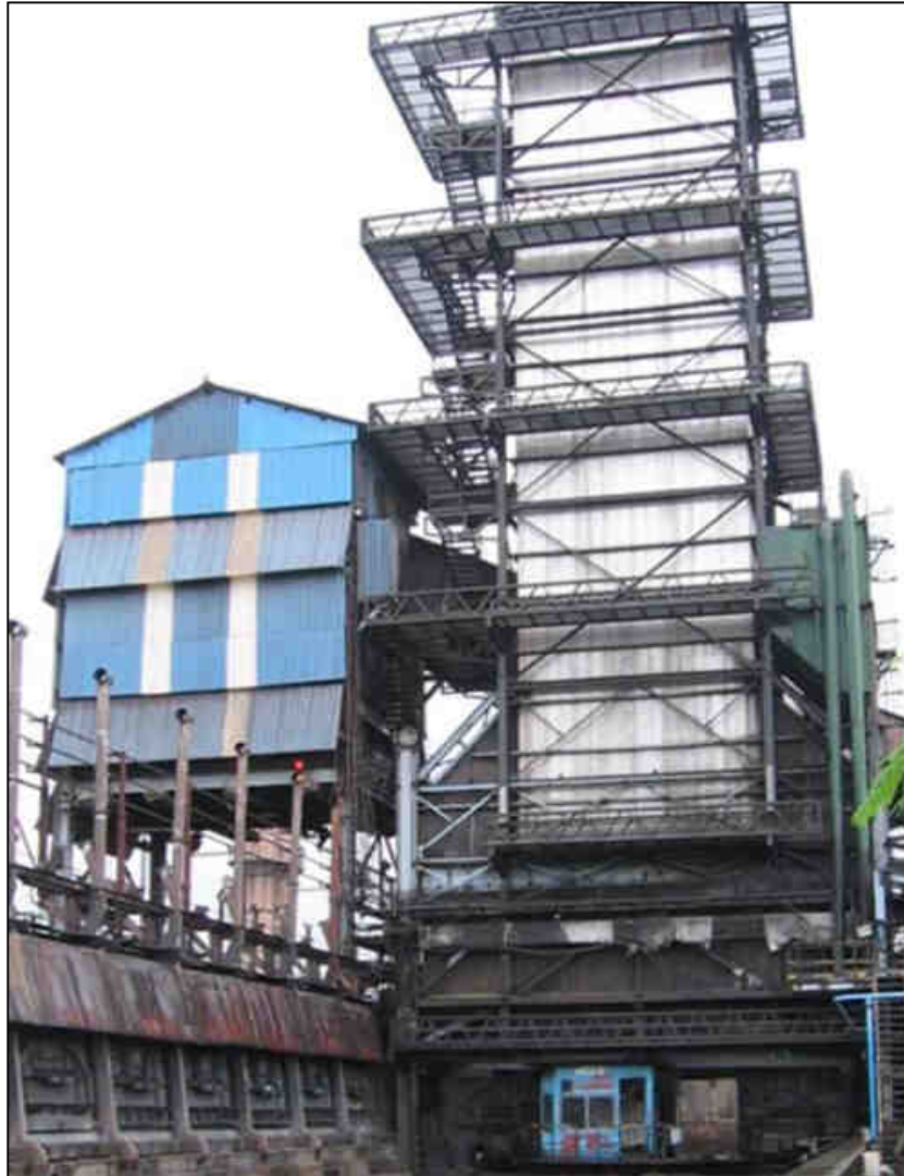
Figure 2.8: Typical quenching tower with quenching car underneath the tower (similar to proposed Market Coke Plant) (Courtesy Sesa Goa Ltd).
