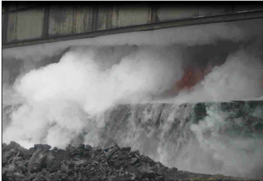
Figure 2.9: Coke cake undergoing quenching (Courtesy Sinosteel).
