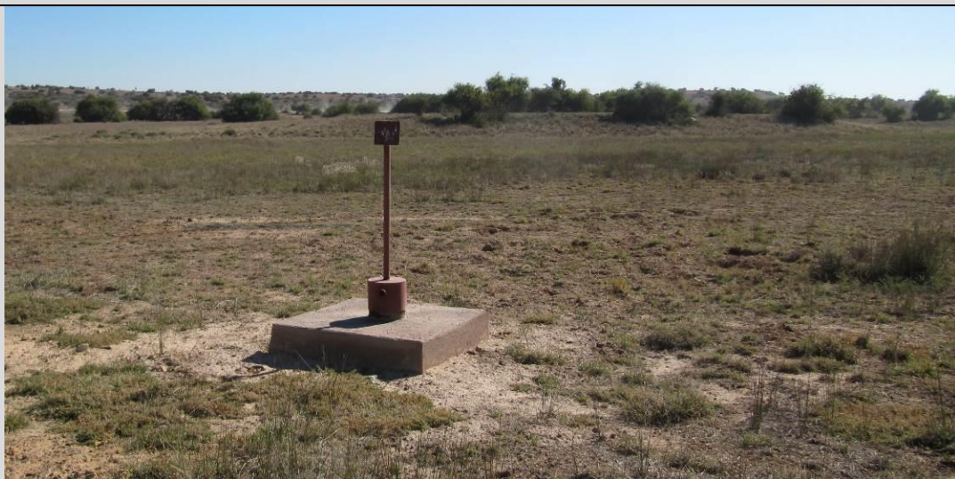
Figure 4: Visual example of borehole, casing and concrete slab required at the LF and KK areas.
