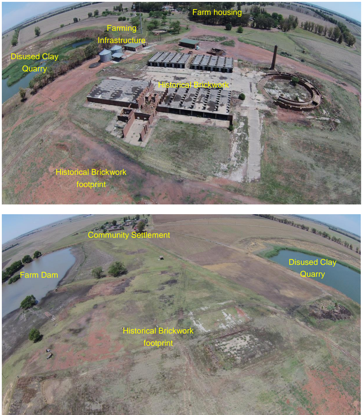
Figure 2: Photographs of the proposed Phosphoric Acid Plant site
