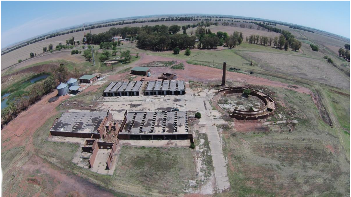
Figure 11: Photograph of the Historical Brickwork
