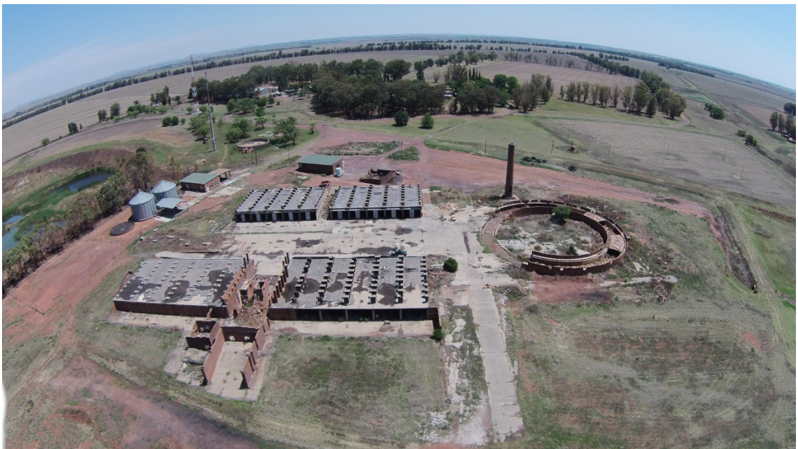
Figure 21: Photograph of the Historical Brickwork
