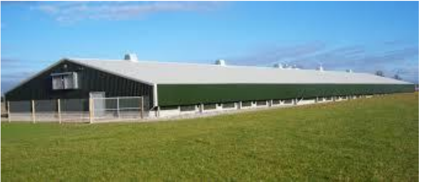
Exterior of the manual ventilated poultry house, with a side foldable plastic cover.
