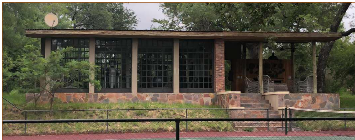
Figure 34: Front view of existing gym (© GAPP).
