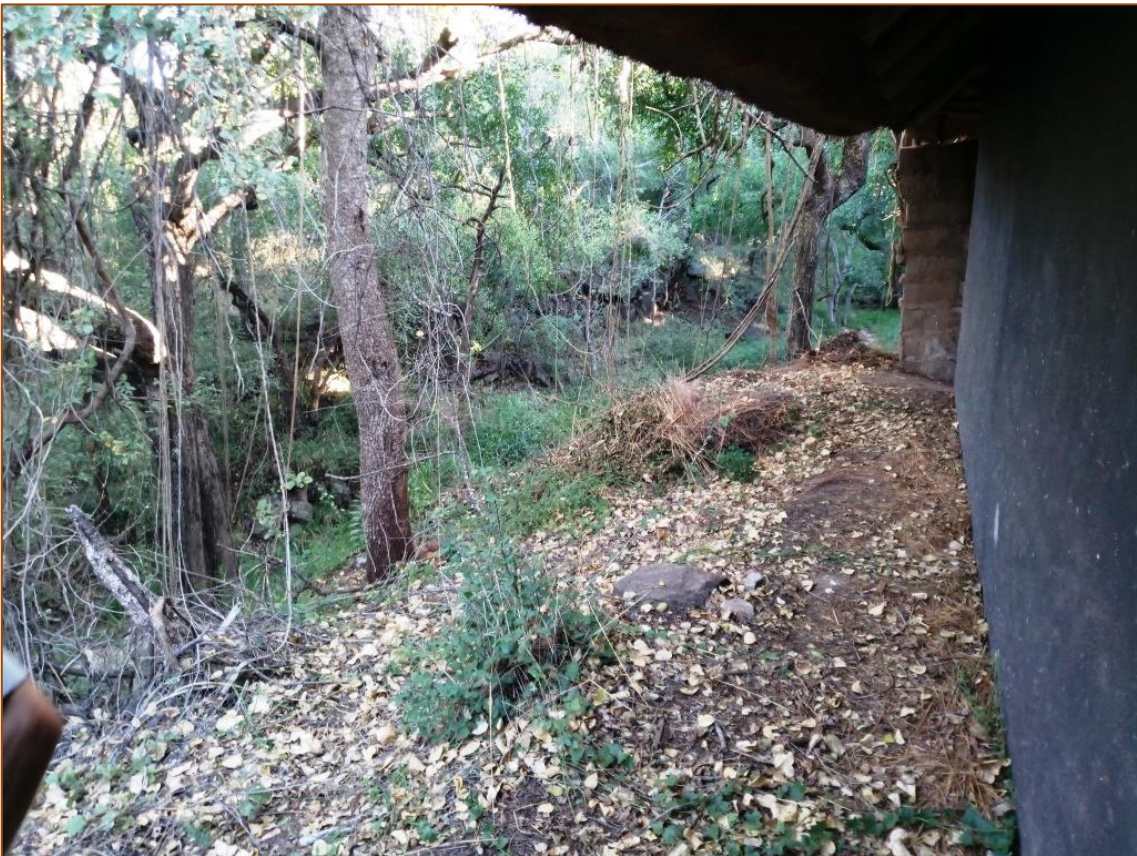
Figure 22: The back of rooms 2 to 6 with the adjacent watercourse to the left (© K Zunckel)
