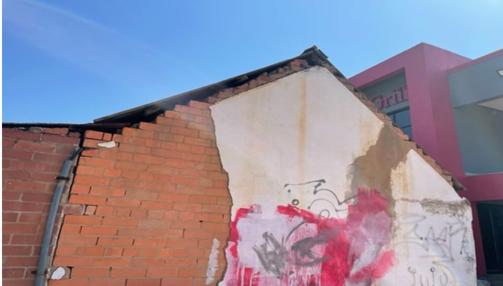
Picture showing the side view of the buildings to be demolished
