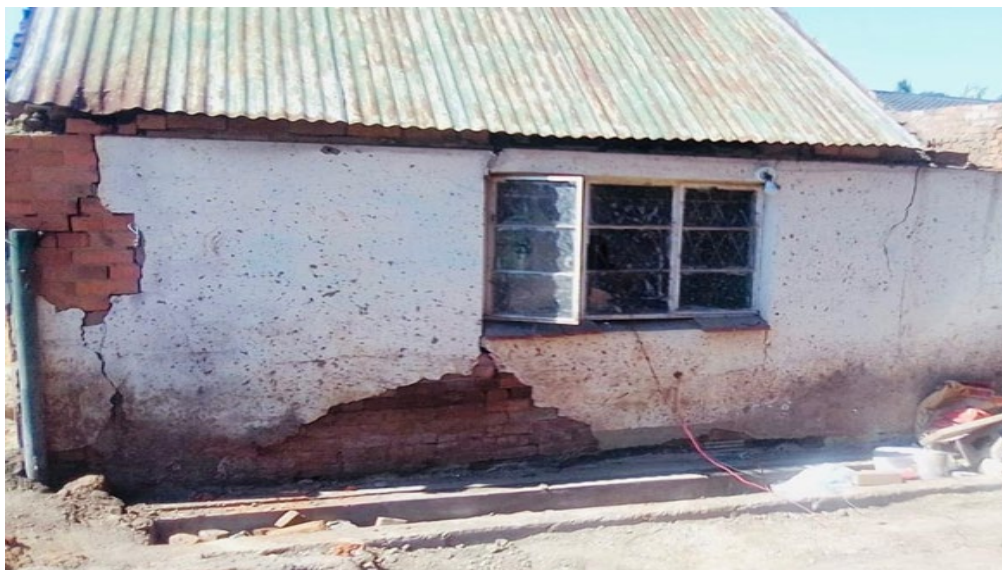
Picture showing the rear view of the buildings to be demolished
