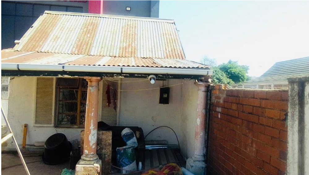
Picture showing the front view of the buildings to be demolished
