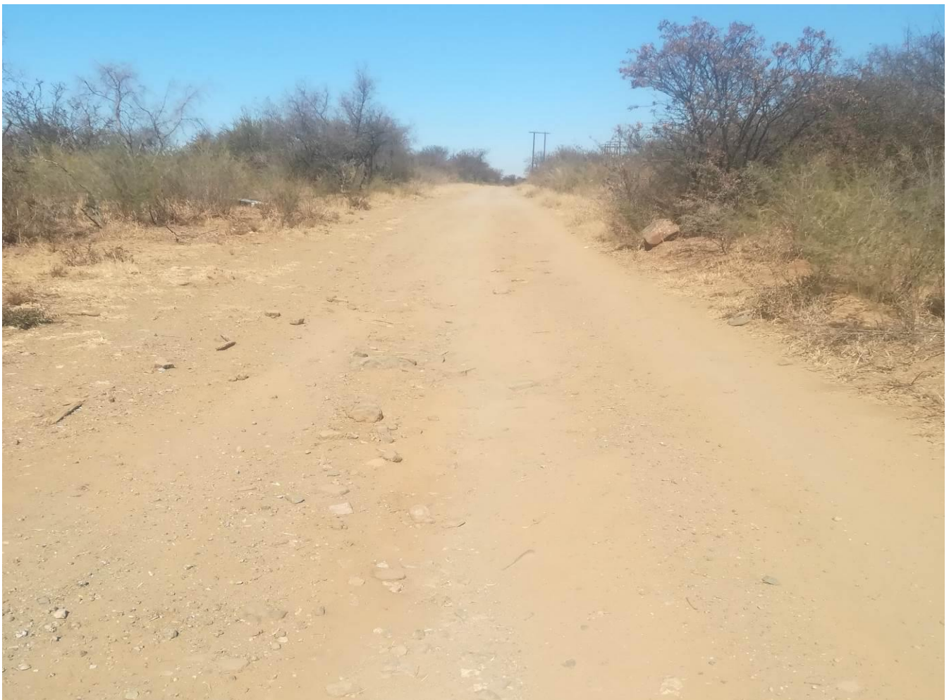
Figure 4: Gravel road next to which the cable will be aligned
