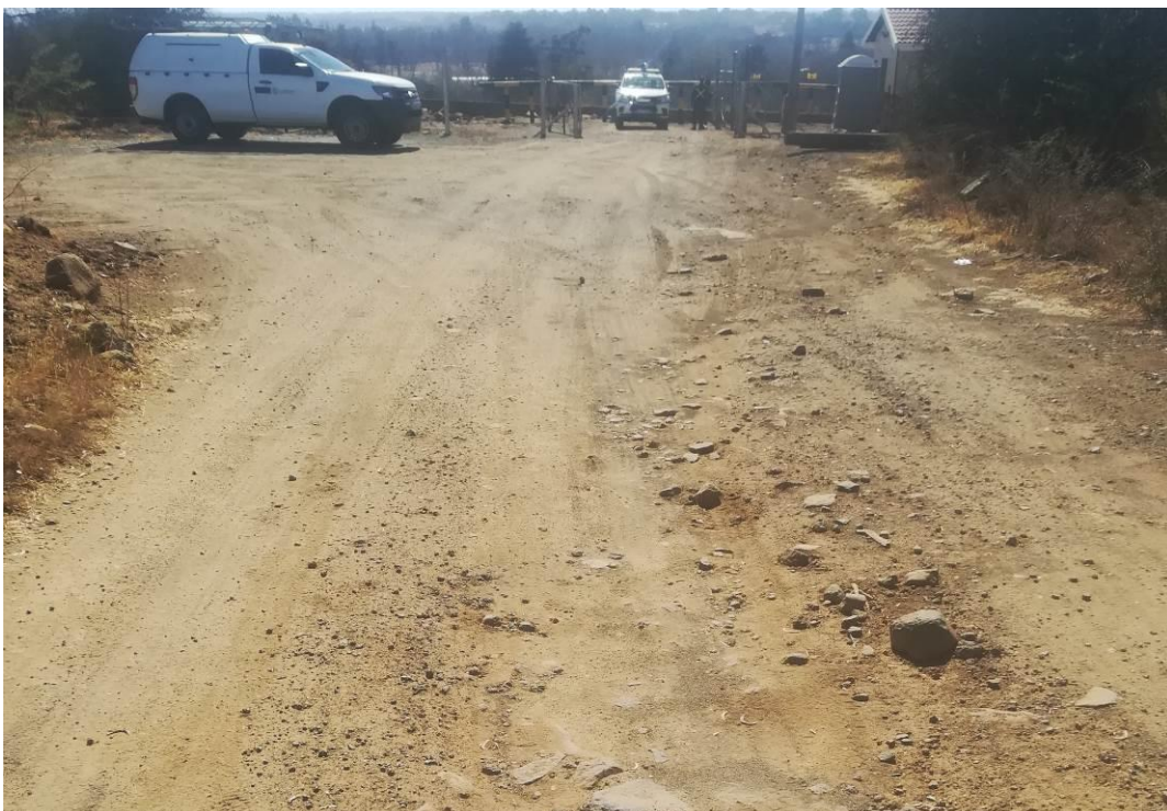
Figure 12: Cable route across the Sasol pump station
