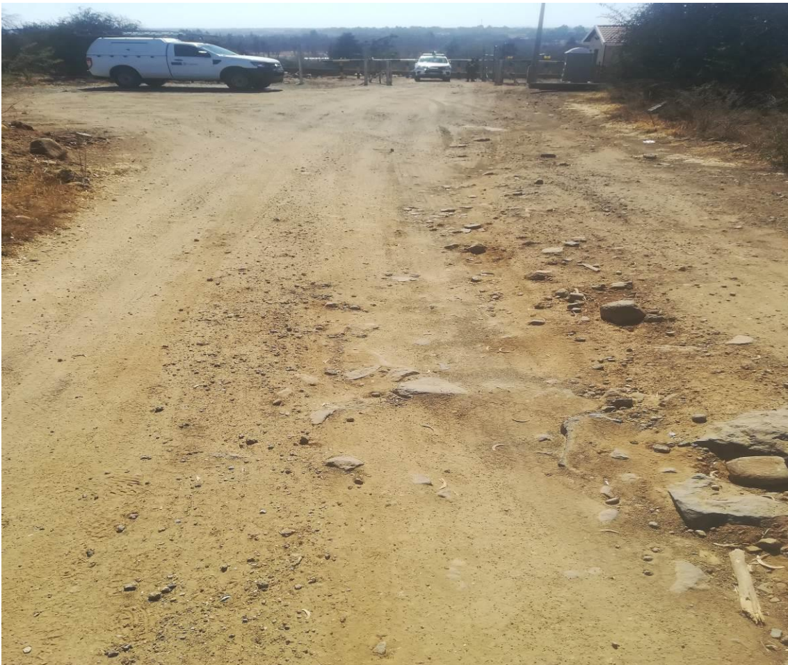
Figure 8: Gravel road to the Sasol pump station
