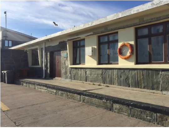
Repair & repainting of Walls.
