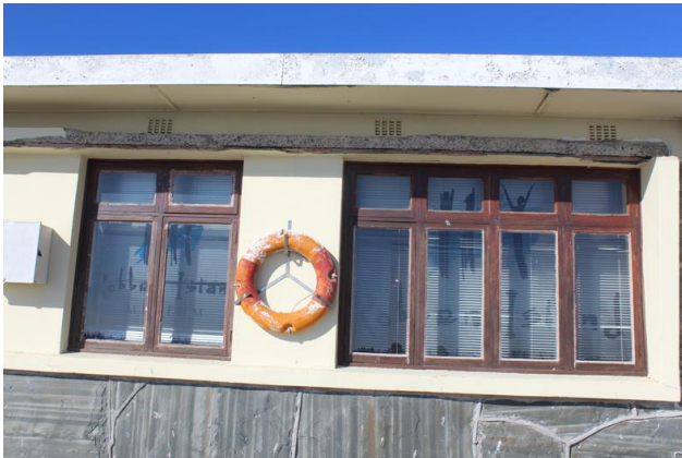
Sand, prime & repaint fascia boards.
