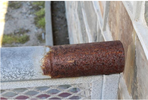
Galvanised rail detail
