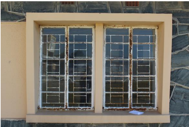
Windows show different levels of deterioration. One would require sandblasting for deep rust removal prior to finishing.
