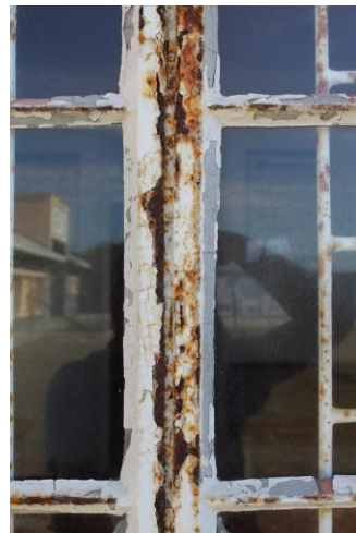
Windows show different levels of deterioration. One would require sandblasting for deep rust removal prior to finishing.
