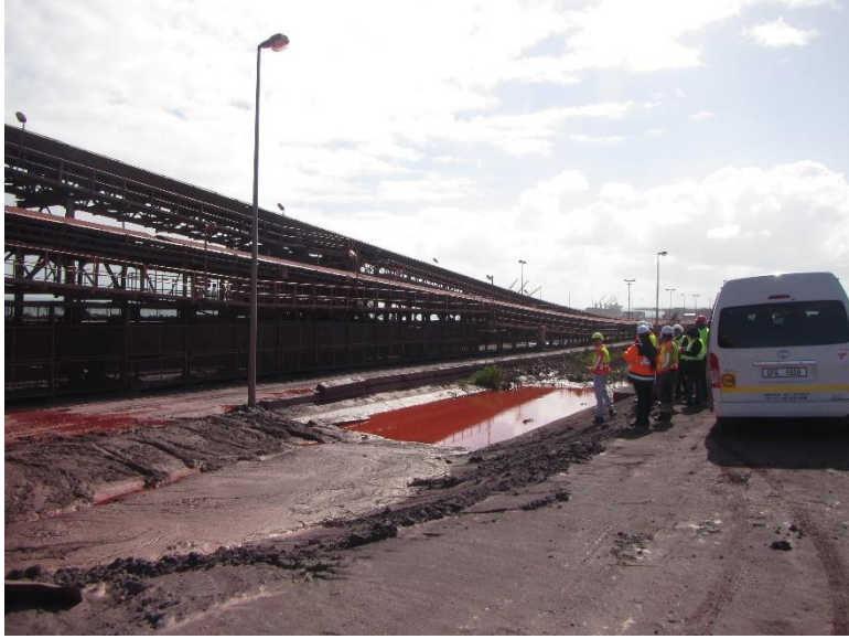
Sludge in the water channel.
