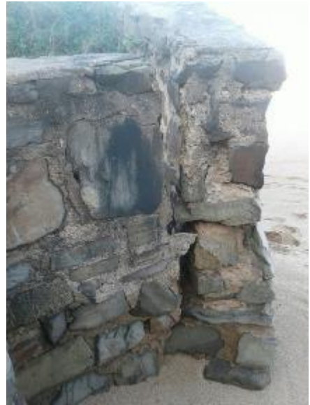
Figure 10 Cross Section View of remaining portion of sea wall.
