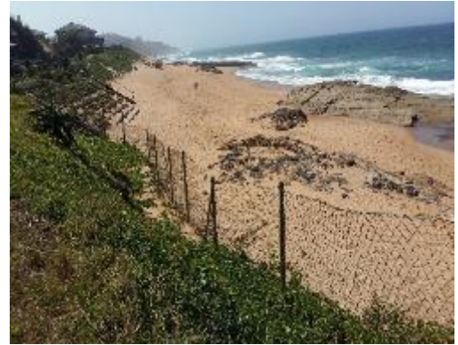
Figure 6 Northern view of sea wall location where wall is to be re-built
