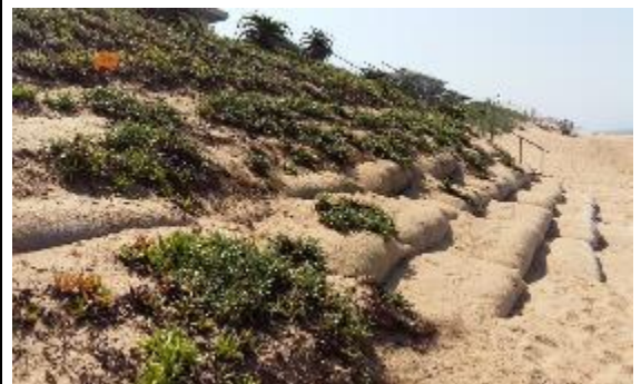
Figure 8 Vegetation cover on sandbags on northern property as example of proposed rehabilitation for sea wall northern tie in area.
