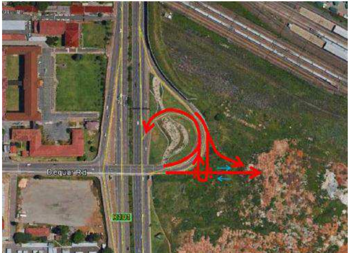
Figure 6: Kgosi Mampuru and Dequar Street Intersection upgrades
