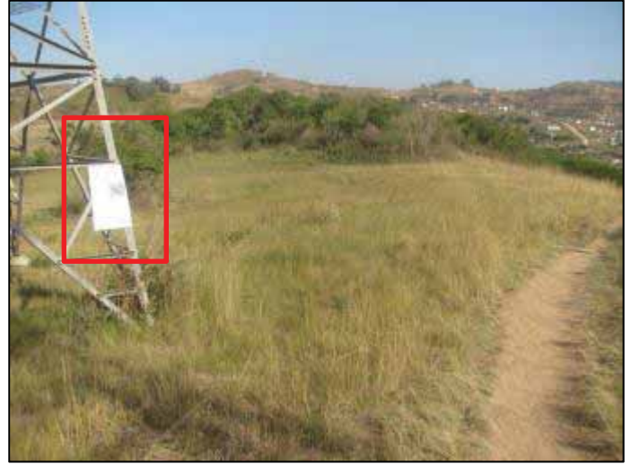
Placement of the notification signboard along the informal footpath leading to the proposed bridge location on the southern riverbank.
