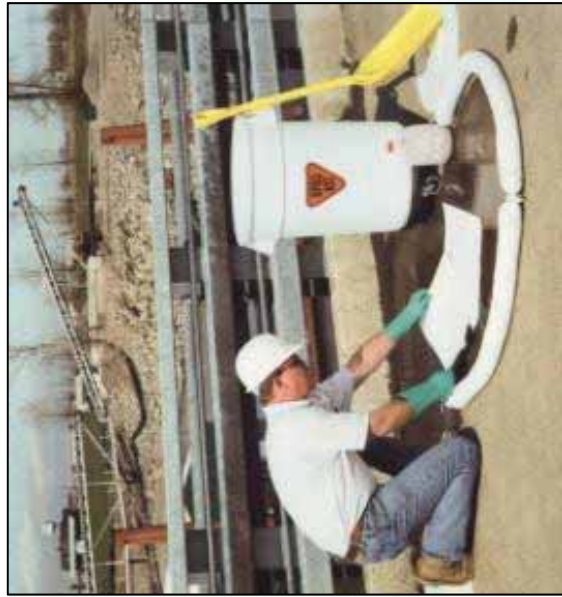
Figure 17: The use of a spill kit during an emergency response to an accidental spill.
