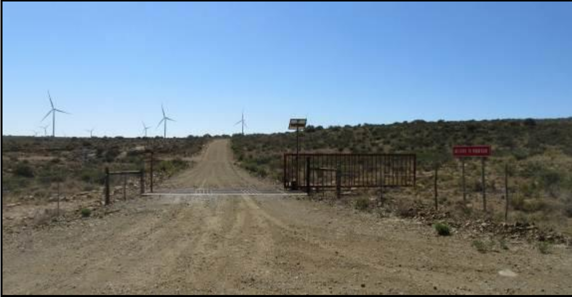
Photograph 3.45: One of two entrances to the Noupoort WEF off the Oorlogspoort gravel road
