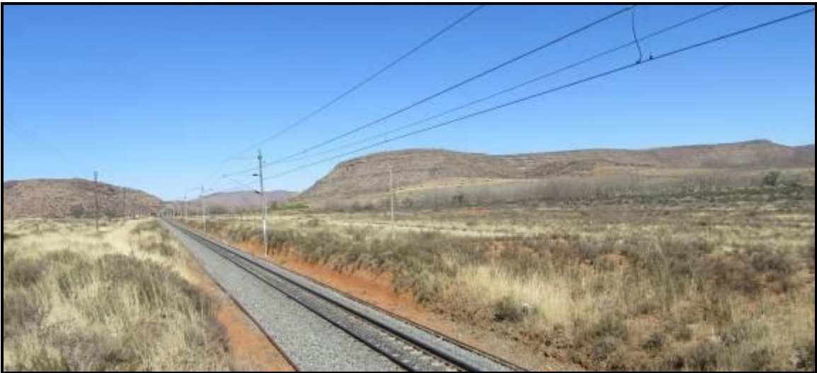
Photograph 3.32: Railway line and 132 kV transmission line on Edendale north of farmyard
