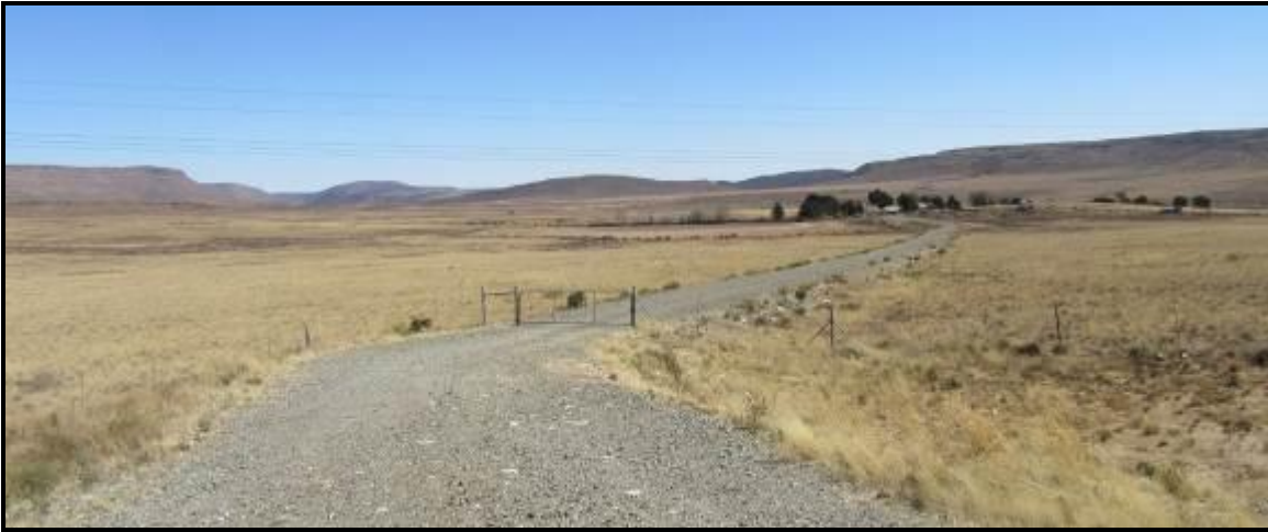
Photograph 3.35: Vrede farm yard and access road off the N9. Note 132 kV cables traversing access road in foreground
