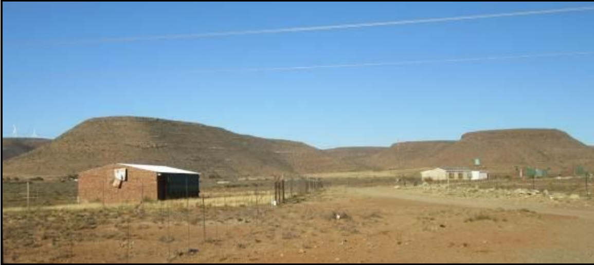
Photograph 3.22: Defunct broiler houses on non-site portion of Hartebeeshoek, seen from the N9
