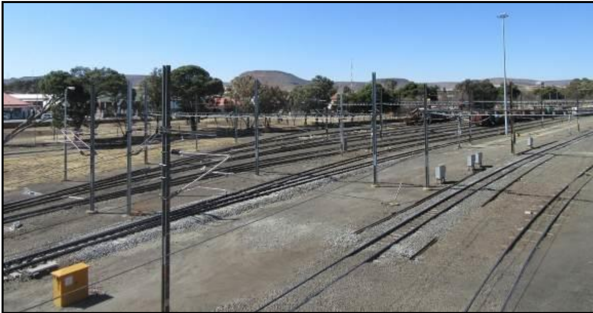
Photograph 3.4: Noupoort station seen from the train bridge in Noupoort
