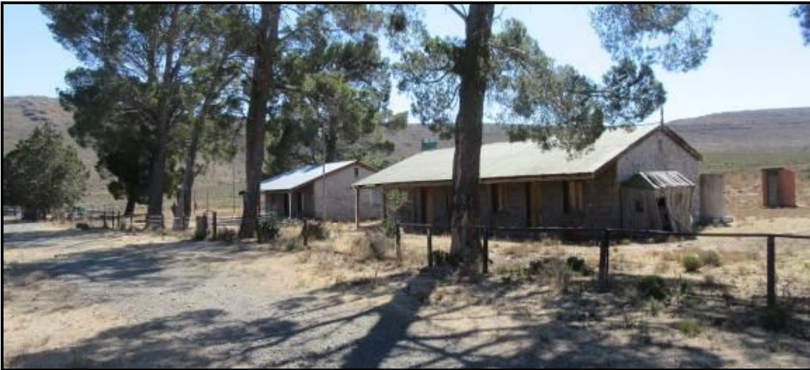
Photograph 3.30: Cottages associated with former De Rust siding on De Rust
