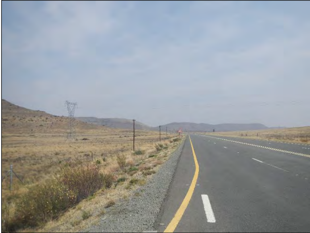
Figure 50: View of some of the existing power lines which are visible from parts of the N9 national route.
