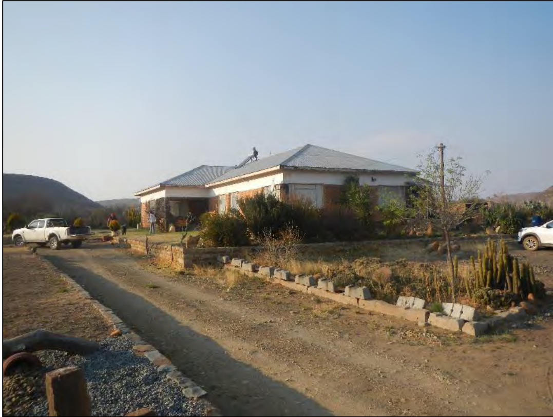
Figure 39: View of the main guestroom / guesthouse facility at The Dairy BnB (VR 28).
