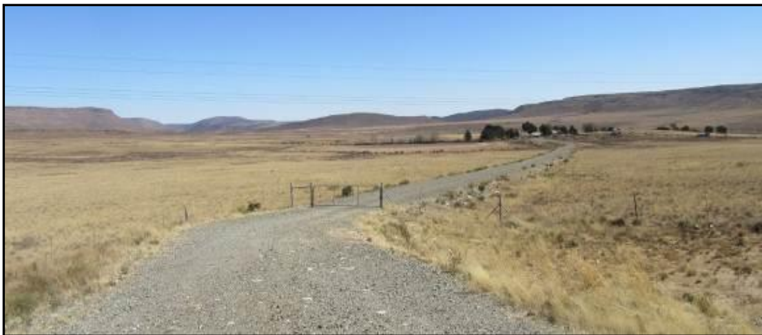
Photograph 7.17: Vrede farm yard and access road off the N9. Note 132 kV cables traversing access road in foreground
