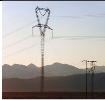
Plate 6-2: Guy line supported steel structures.
