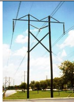
Plate 6-4: Multi-pole structures such as H-towers or K-towers.
