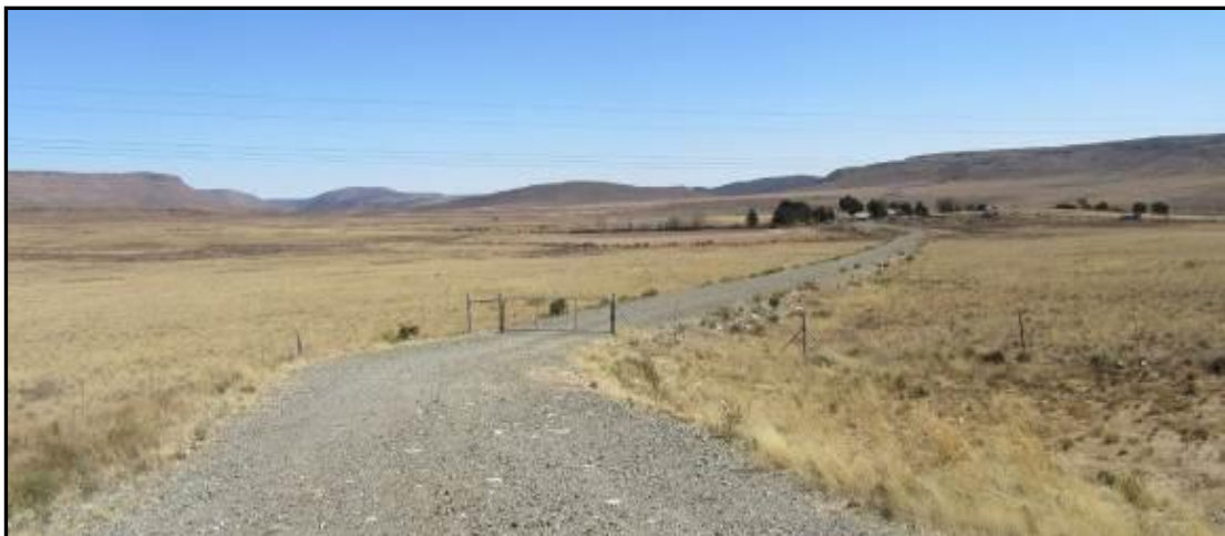
Photograph 7.17: Vrede farm yard and access road off the N9. Note 132 kV cables traversing access road in foreground
