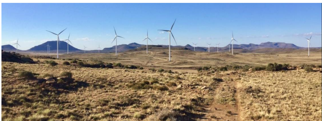
Figure 8.17. The nearby established Noupoot wind farm reflects how the San Kraal landscape will change.
