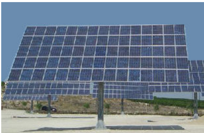
Figure 2.3: Illustration of a tracking photovoltaic panel
