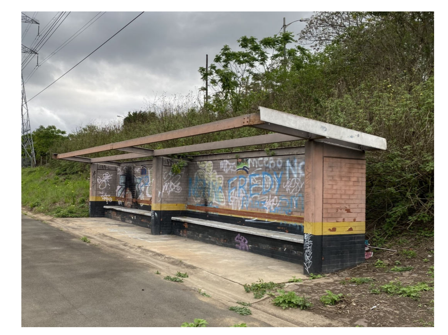
3. EXISTING PUBLIC SEATING 2 (UNLAWFUL WORK)
