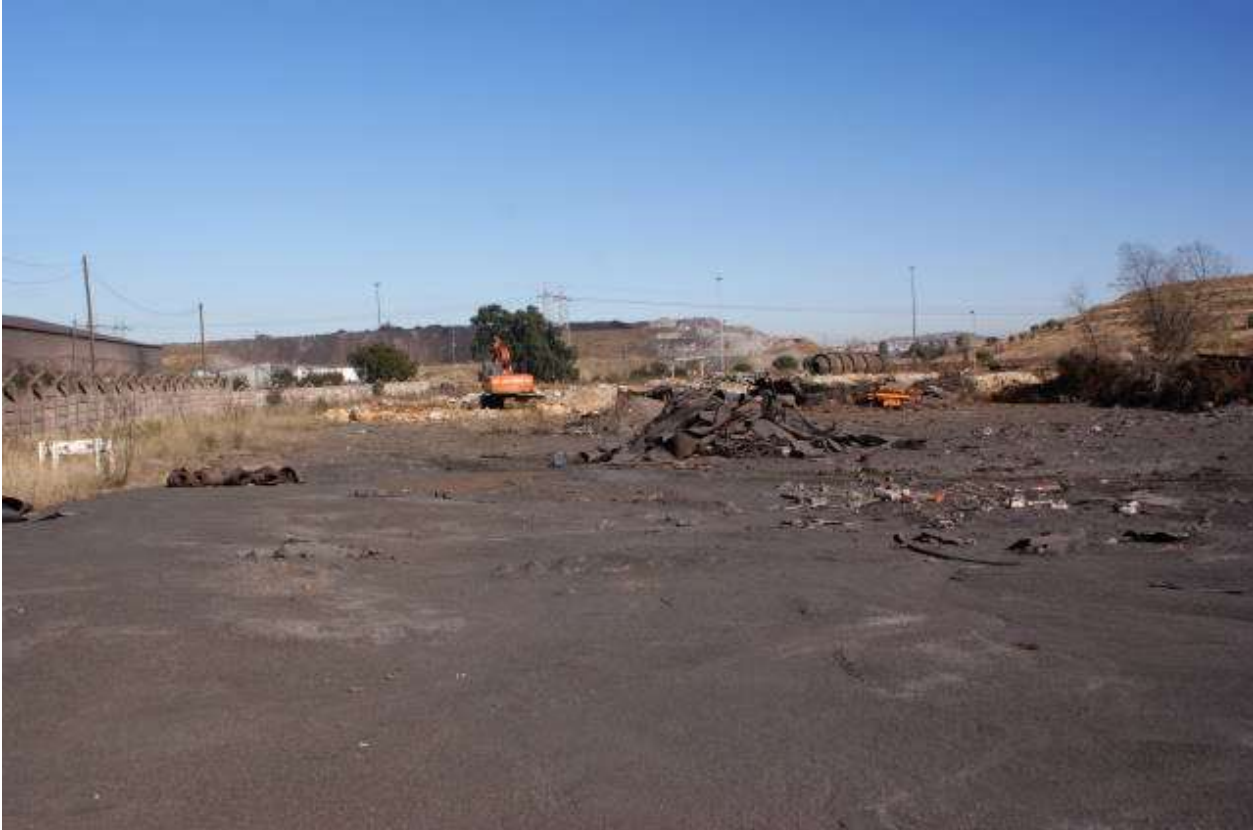
Plate 1: View of the site for the Electrical Co-generation Plant (DRI plant to the left)
