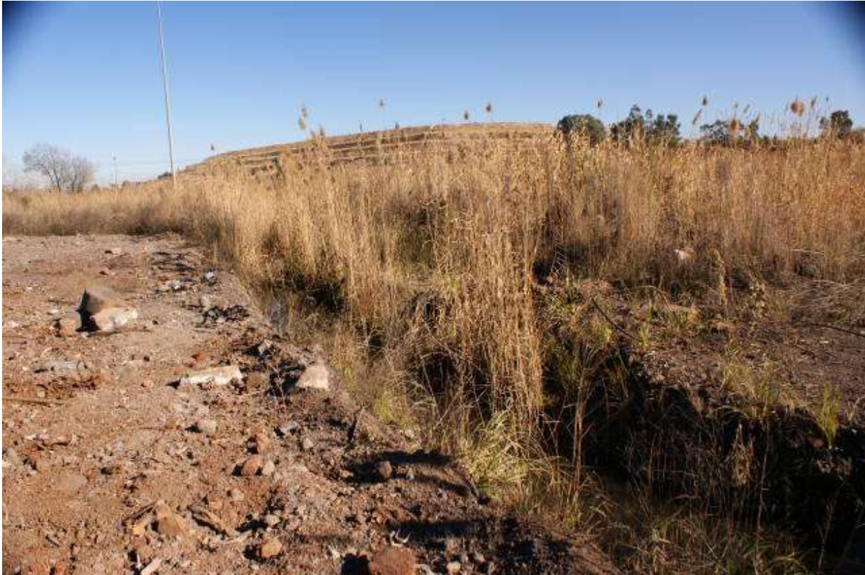
Plate 3: Storm water channel on the Electrical Co-generation Power Plant footprint
