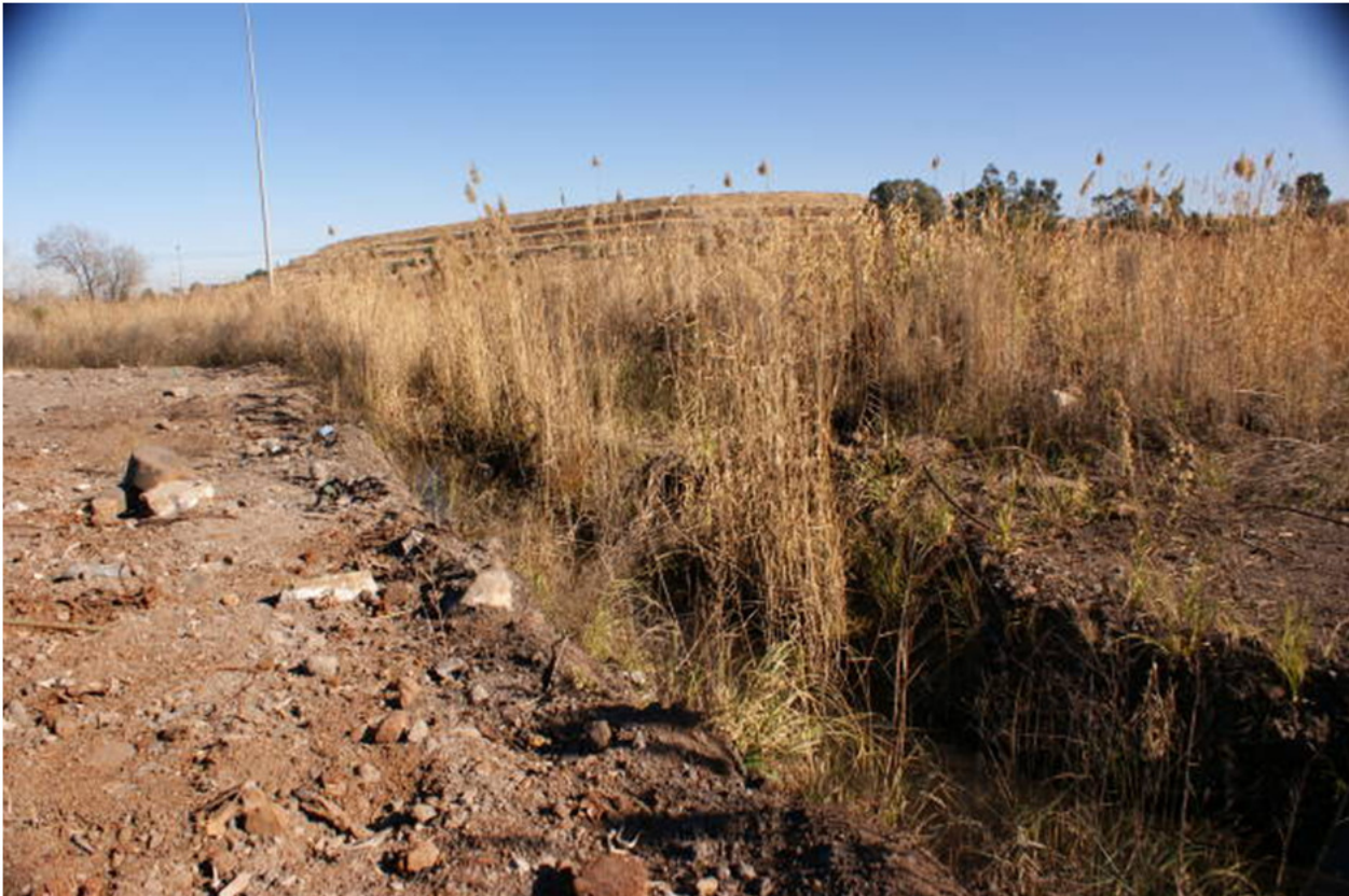
Plate 4: Storm water channel on the Electrical Co-generation Power Plant footprint
