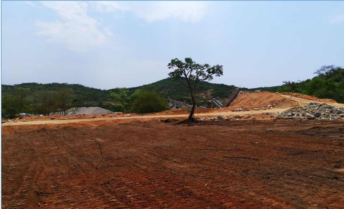
Figure 15: Shows the type of soil observed during the site assessment of the proposed area.
