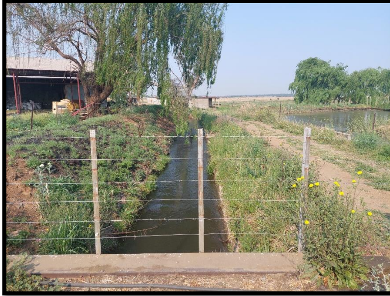
Photo 4: Open-on-top cement canal on site
