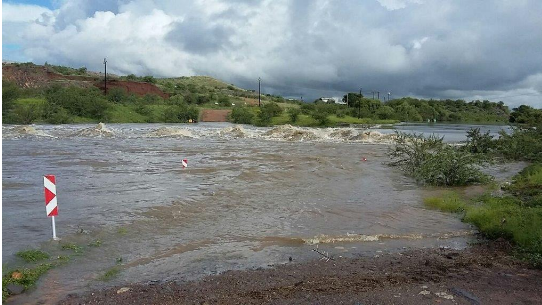
Figure 3-6: Driekuilspruit river crossing below the Driekuilspruit Dam wall during the 2017 flood
