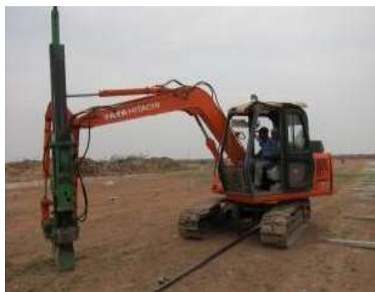
Figure 2.1.: Rammed Pier foundations preferred for the Scuitdrift Solar Energy Facility Figure 2.2.: Installation of Rammed Pier foundations
