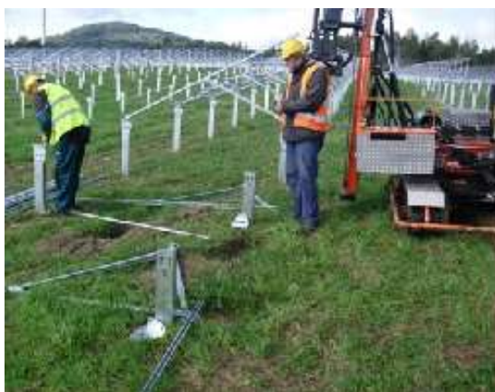
Figure 2.1.: Rammed Pier foundations preferred for the Scuitdrift Solar Energy Facility Figure 2.2.: Installation of Rammed Pier foundations
