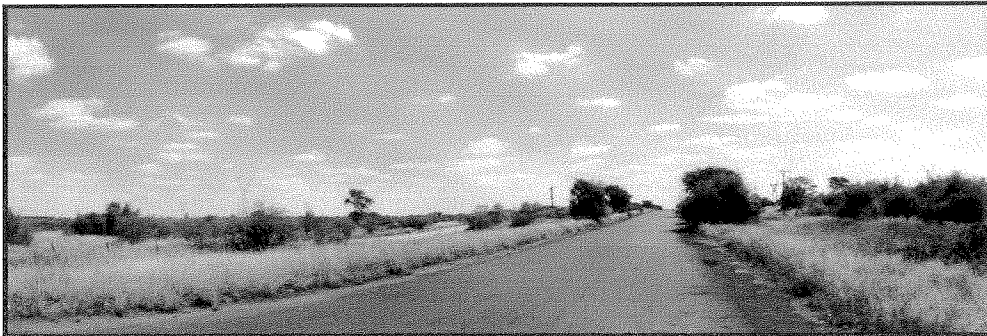
Figure 6: Existing power line corridors (background) within the study area.
