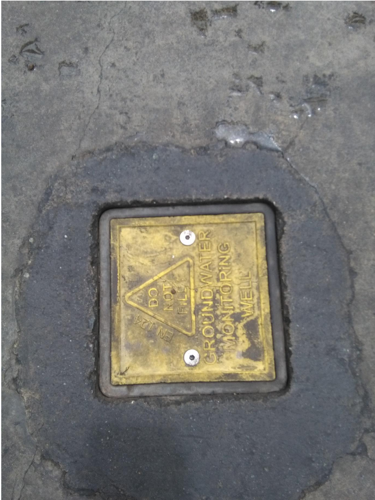
Figure 7-4 Groundwater monitoring well that was first installed in 2014 which African Group Lubricants currently monitors for contamination.
