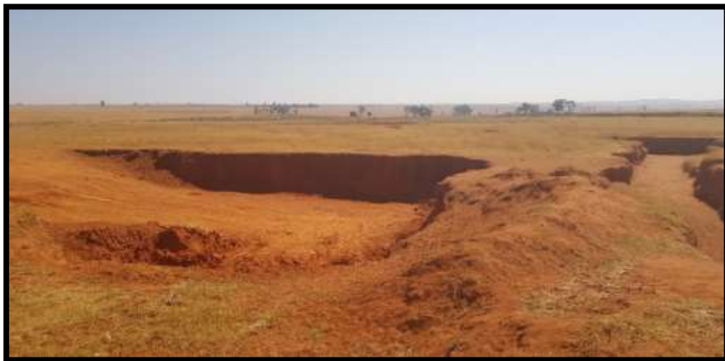
Photograph 4. Excavation of soil
