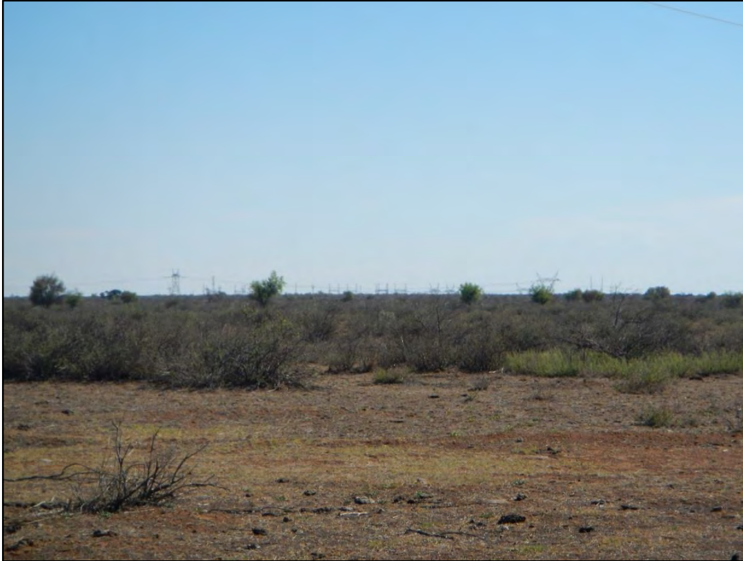
Figure 12: View from within the application site showing the Mookodi MTS which is located north-east of the application site as well as the 400kV power line that bisects the northern section of the visual assessment zone.
