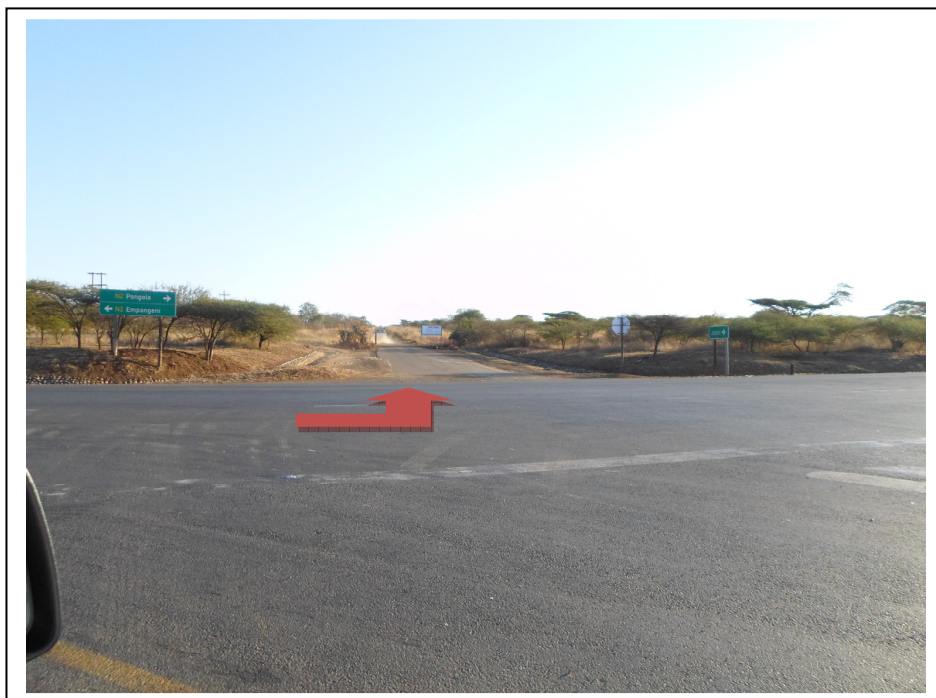
Figure 7: Senekal 1 existing access road off the N2
