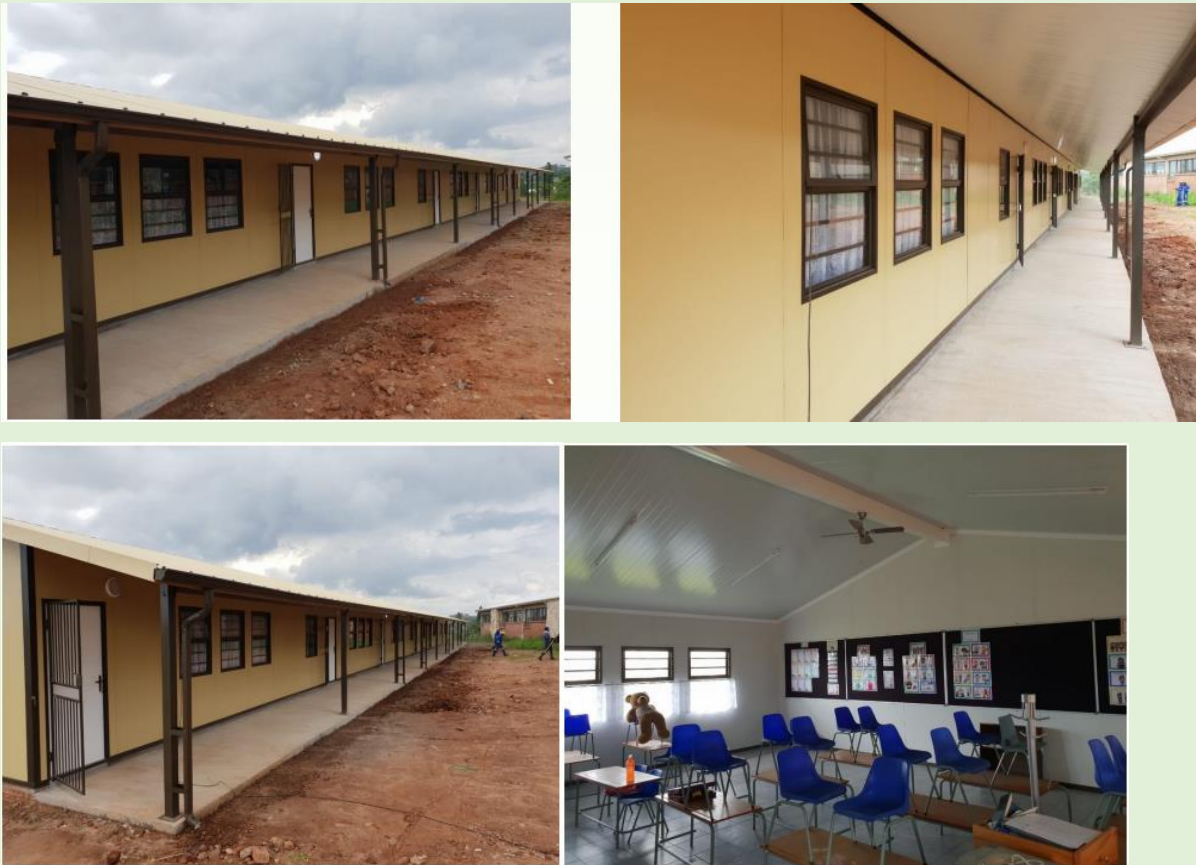
Figure 3: Typical examples of pre-fabricated classrooms
