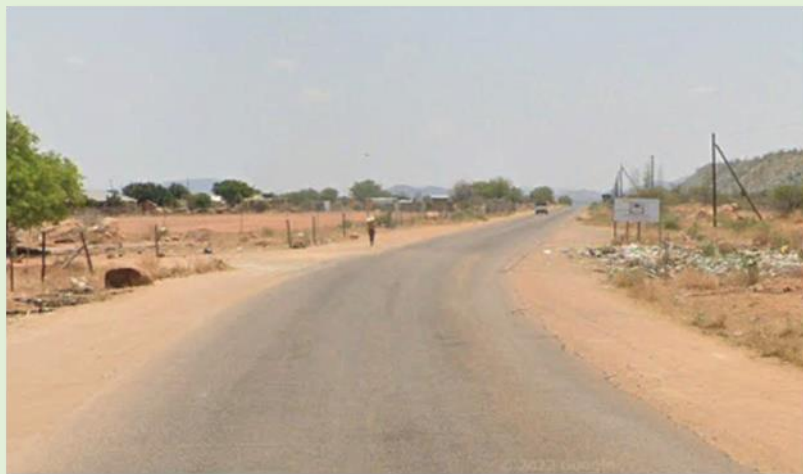
Figure 18: Bakenberg Road (Zutari, 2023)
