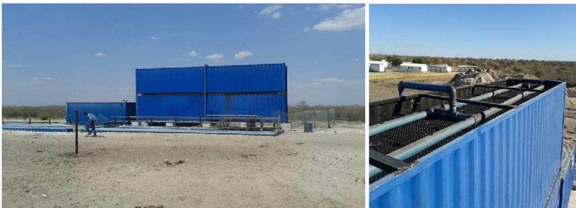
Figure 6: 180 m 3 /day Containerised STP - Discovery Metals, Botswana (31481508)
