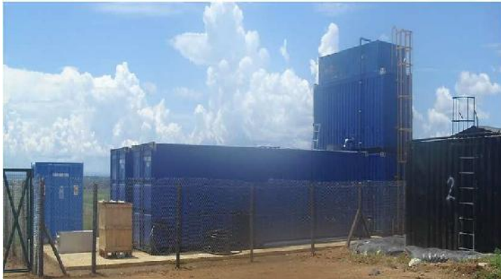
Figure 8: 45m 3 /day Containerised STP - Tullow Oil, Uganda (31481484)
