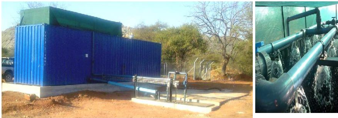
Figure 5: 50 m 3 /day Hybrid STP - BCL Mining, Botswana (31481514)
