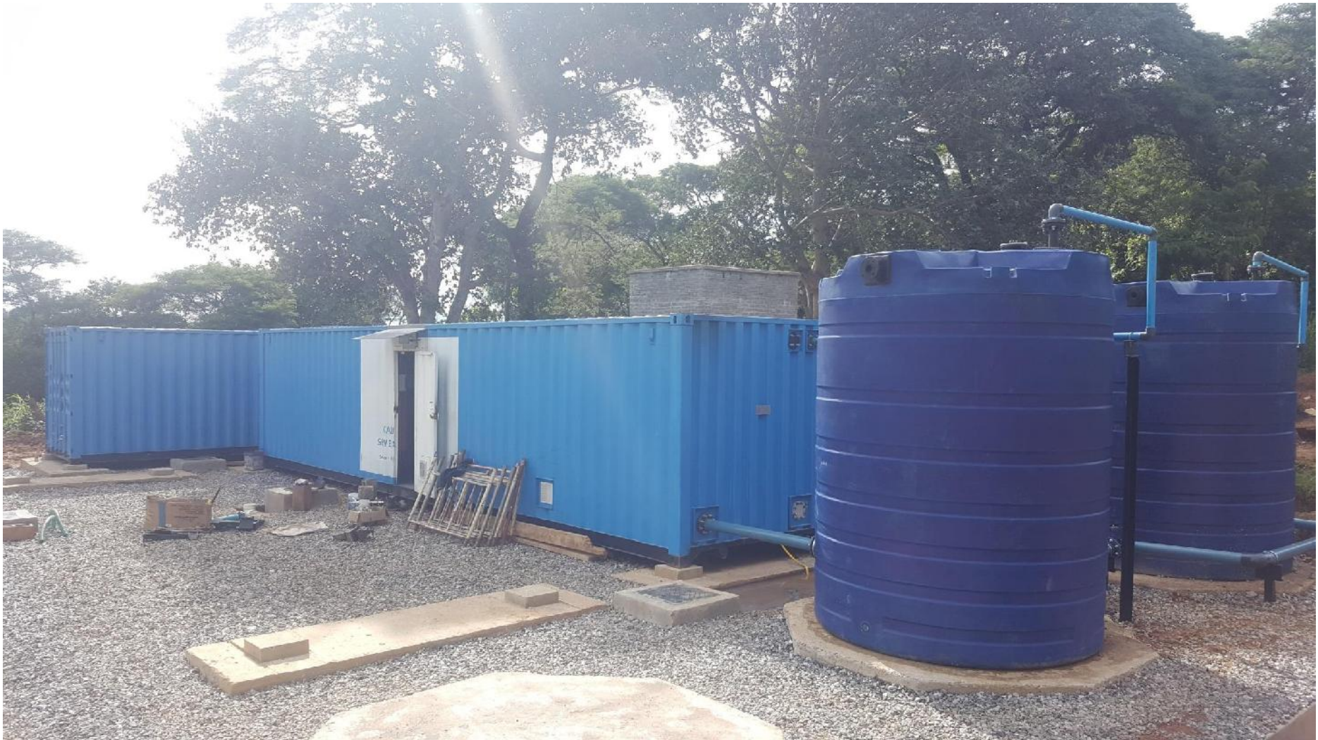
Kafubu Water and Sanitation Improvement Project - D&B
