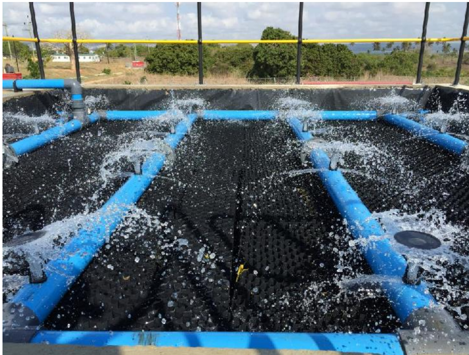
Figure 5: Water distribution in a trickling filter
