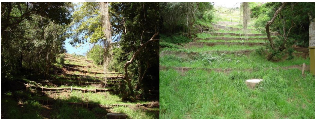
Example of soil erosion protection by means of silt fences and logs
