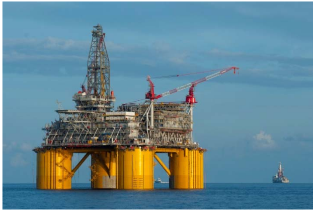
Figure 3.2a: Photograph of a semi-submersible drilling unit (Source: Shell).
