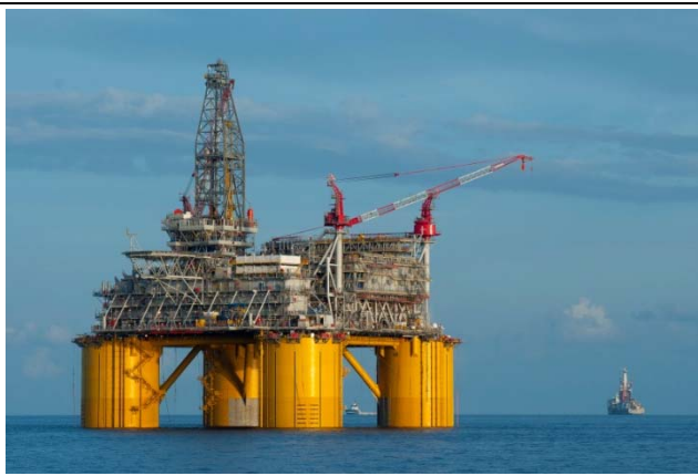
Figure 2a: Photograph of a semi-submersible drilling unit (Source: Shell).
