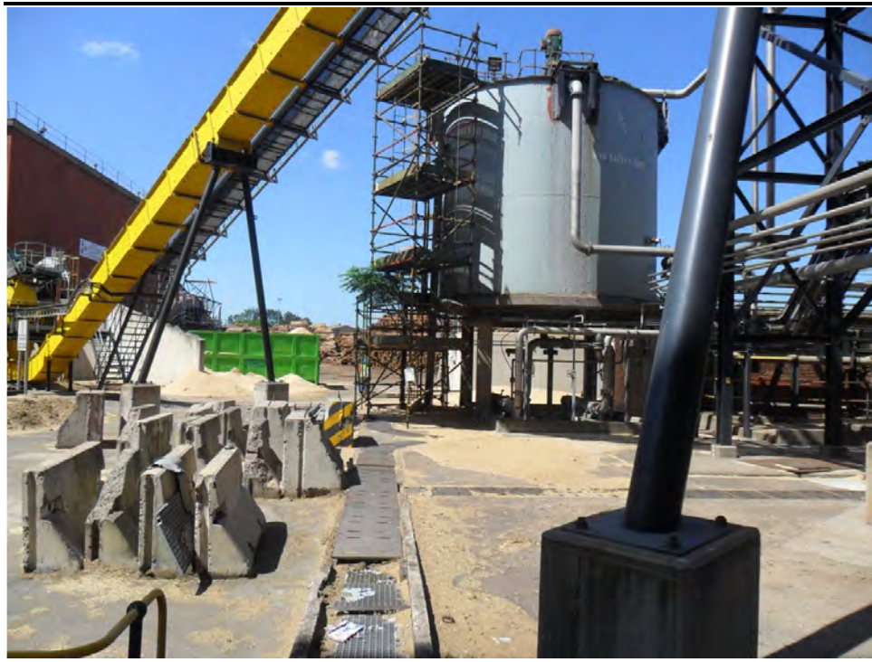
Figure 1.6 View from the HFO tanks facing north-east
