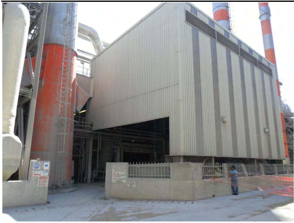
Figure 1.9 View from the HFO tanks facing south-west
