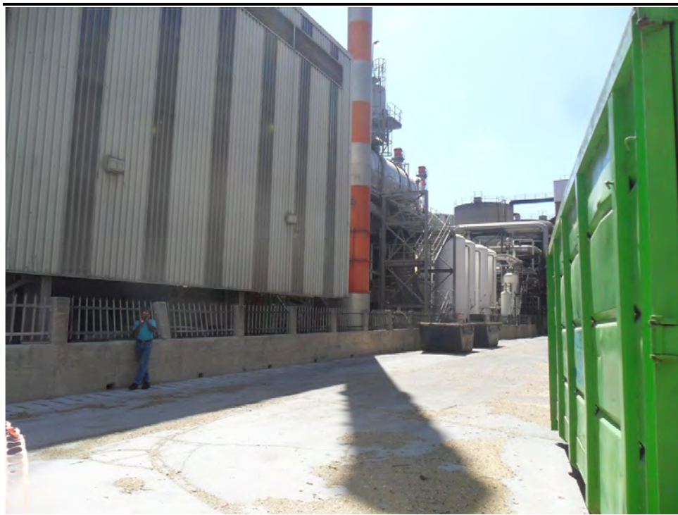
Figure 1.5 View from the HFO tanks facing west
