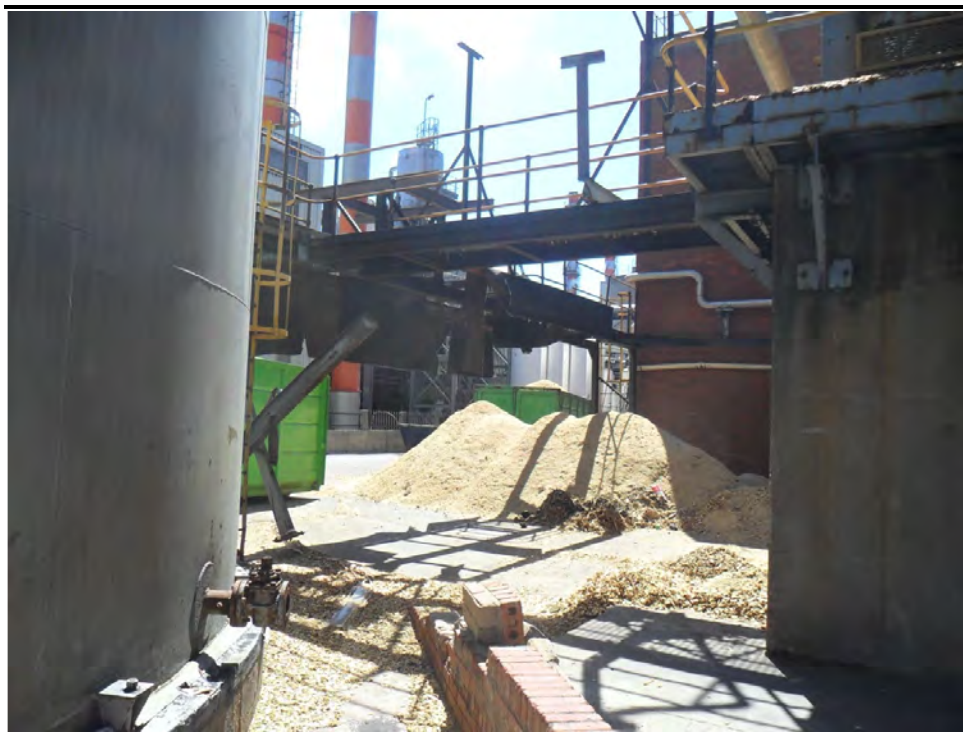
Figure 1.7 View from the HFO tanks facing north-west
