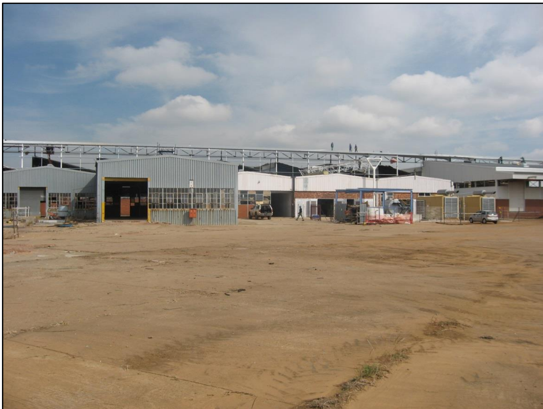
Figure 8: View of a section of the existing old plant.
