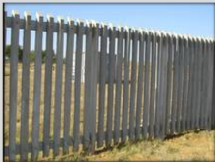
Figure 3 : Concrete pallisade fence – For the cemetery boundary wall
