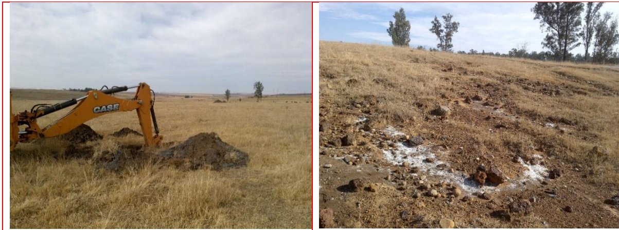
Figure 2-6: Photographs of the CWA (Date: 18/03/2020) showing the variable surface conditions
