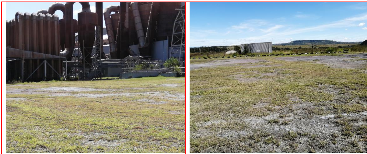
Figure 2-10: Photographs of the Historic Power Station Cooling Ponds (Date: 18/03/2020)
