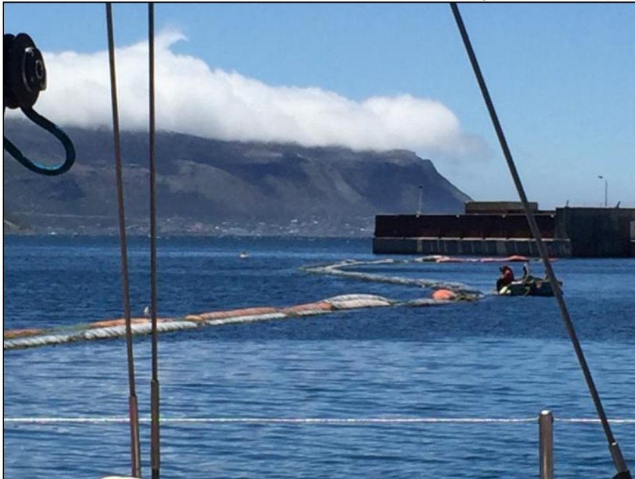
Figure 21: Current breakwater at Simon's Town Marina
