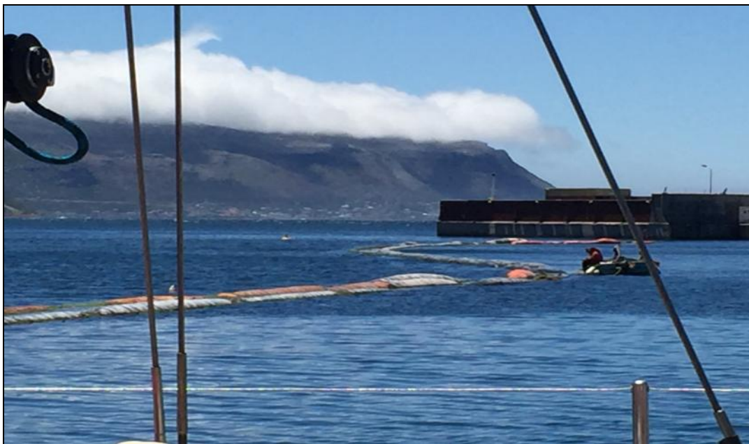
Figure 3: Breakwater structure currently present at the Marina
