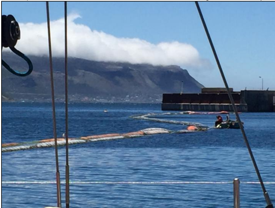
Figure 30: Current breakwater at Simon's Town Marina
