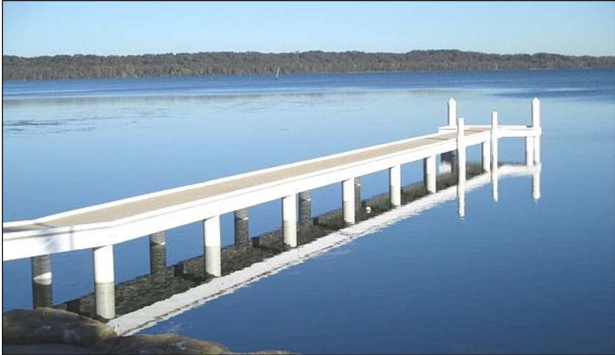
Figure 19: An example of a jetty installed on piles
