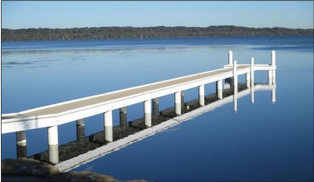
Figure 12: An example of a jetty installed on piles
