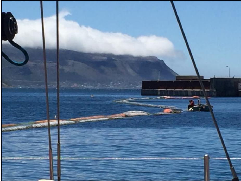
Figure 14: Current breakwater at Simon's Town Marina
