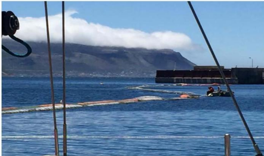
Figure 3: Breakwater structure currently present at the Marina
