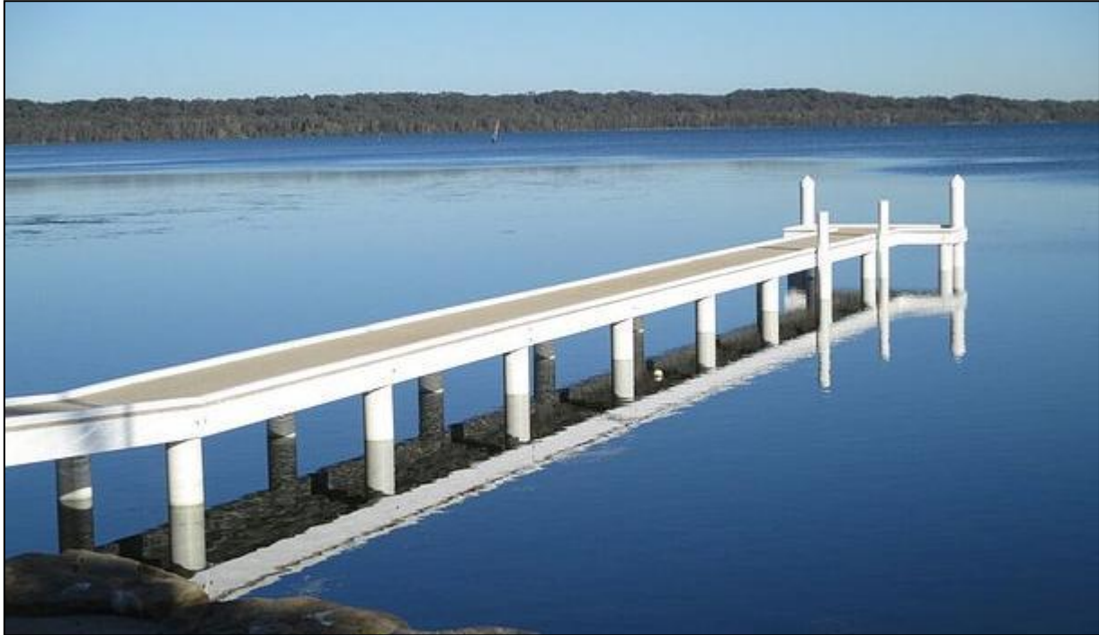
Figure 28: An example of a jetty installed on piles
