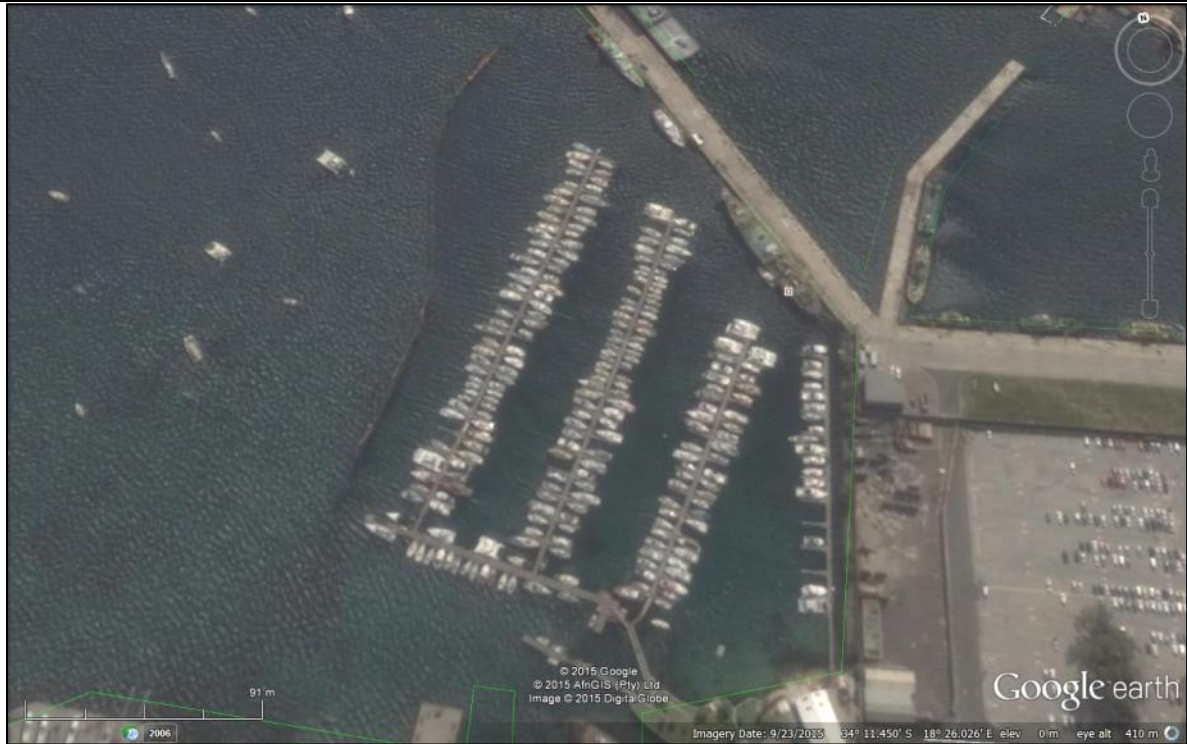
Figure 16: Current breakwater installed at Simon's Town Marina
