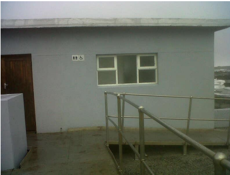
fig. 6 North Elevation of Pump House
