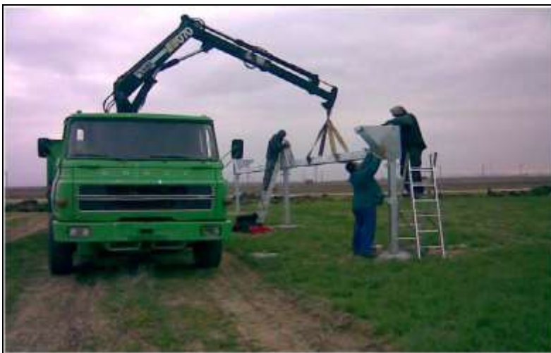
Figure 2.12: Mounting of the frame for the PV panels (Courtesy of Igeam, 2011)
