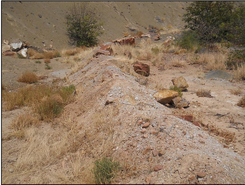
Figure 8. Example of a toe berm.
