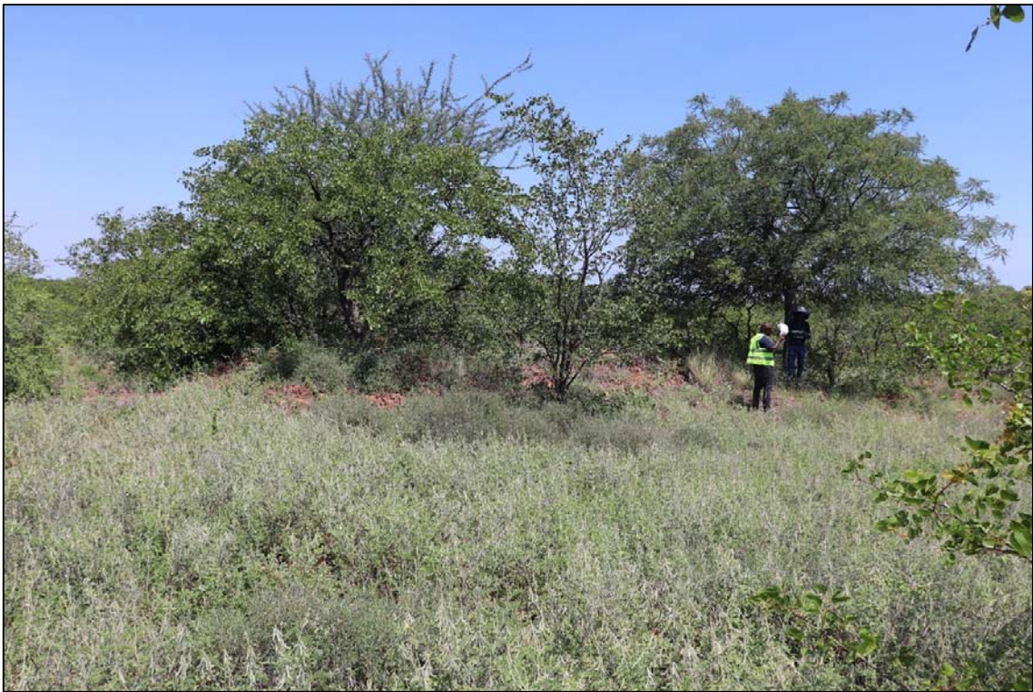
Figure 6: Cleared area that resulted from the construction of the gravel road
