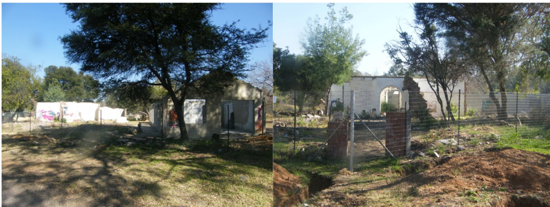
Demolished mine houses surrounded by fence
