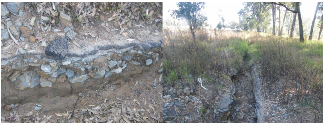
Trench next to the derelict road on site
